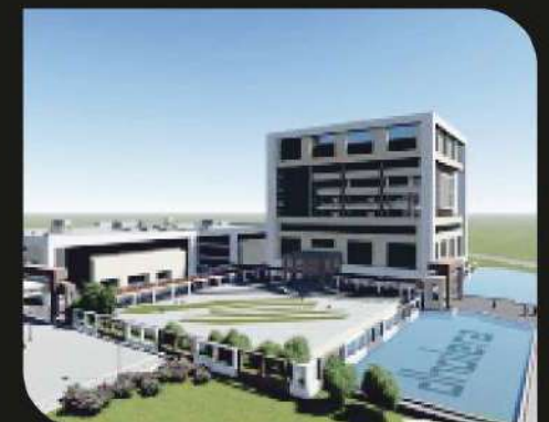
Dholera ABCD Building Single Window Clearance
